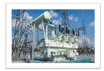
Alpha-1 Fluid. Alpha-1 Fluid adds a significant safety margin to equipment designed for use with standard, more flammable oils. Alpha-1 mixes well with PCB fluids, Wecosol, mineral oil and vegetable oils. Retrofilling with Alpha-1 Fluid is usually a simple matter of draining, flushing and then refilling the transformer (1). Contact Soltex for more information regarding retrofilling procedures with Alpha-1 Fluid.
