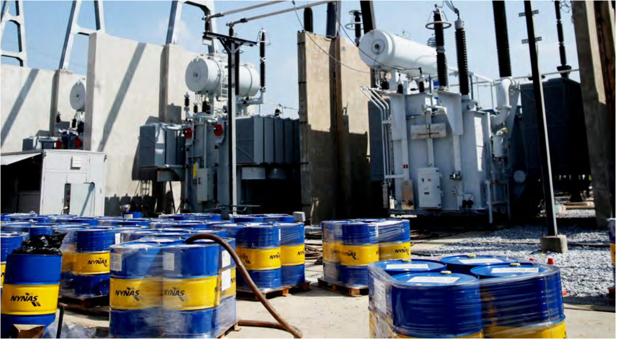
Fig 2: Transformer Oil Used in Power Transformers
