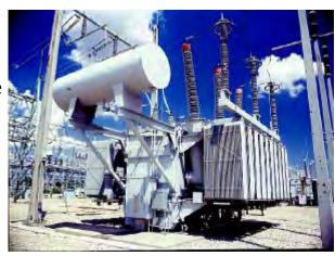
Alpha-1 Fluid. Alpha-1 Fluid adds a significant safety margin to equipment designed for use with standard, more flammable oils. Alpha-1 mixes well with PCB fluids, Wecosol, mineral oil and vegetable oils. Retrofilling with Alpha-1 Fluid is usually a simple matter of draining, flushing and then refilling the transformer (1). Contact DSI for more information regarding retrofilling procedures with Alpha-1 Fluid.
